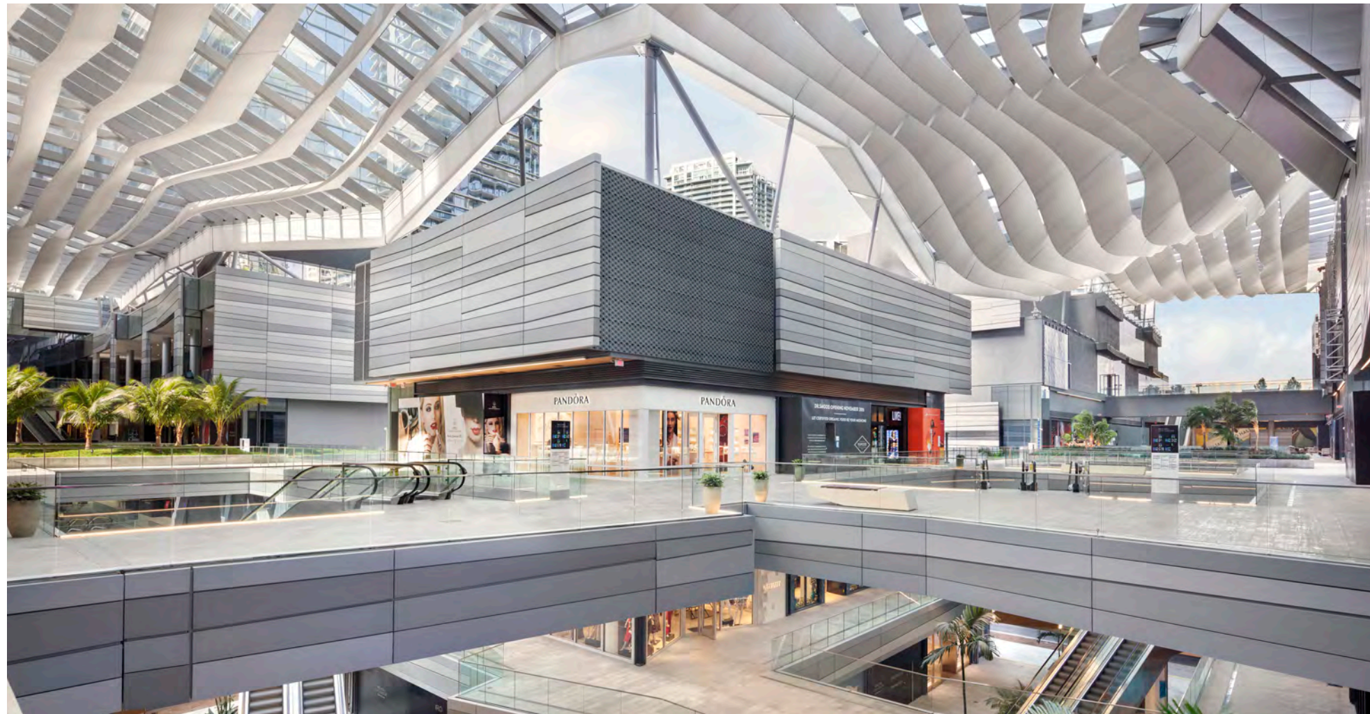
Brickell City Centre, Miami, Florida
